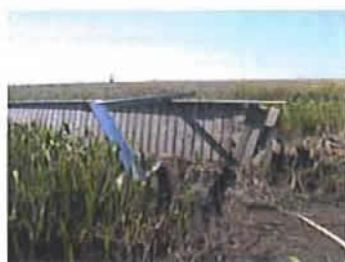
Figure 3. The entry sign, and some boardwalk, neither in a useful position. Photo: Tiffany McFalls.
